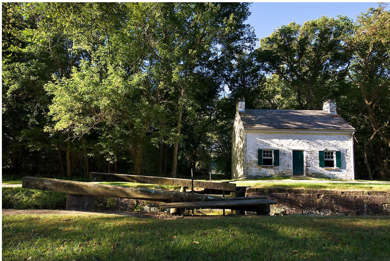
Fig 3. Lockhouse 22 in the C&O Canal National Historical Park. Photo courtesy C&O Canal Trust.
